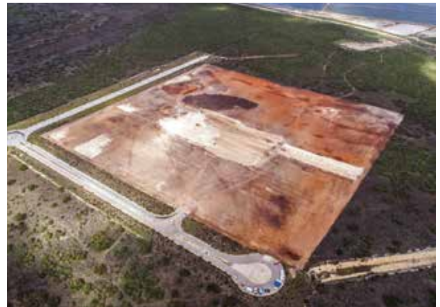
▲ The 20 ha Port of Ngqura Tank Farm site cleared of vegetation in preparation for bulk earthworks.
