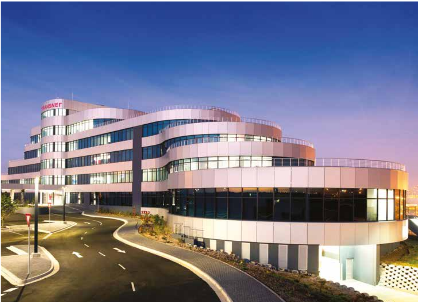
▲ eMendi, the state-of-the-art port administration building.
