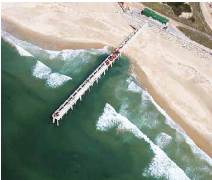
▲ The port is the first port in the world to have a fixed jet pump sand bypass system. This computer-controlled system mimics the natural longshore drift of sand along the coast.
